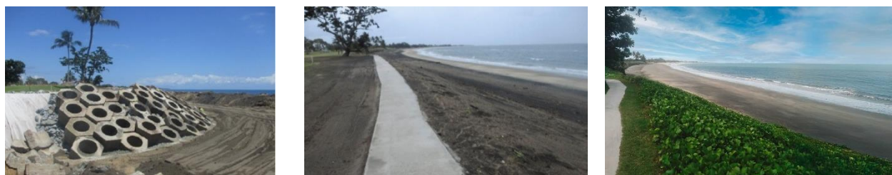
Figure 3: Left: During construction utilising Seabee units, Middle: After construction, Right: Dune development post works (ICM, 2017)
