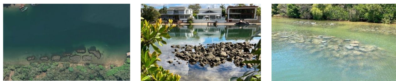
Figure 10: Left: Drone image of new constructed Oyster reefs, Middle: Land based image of Oyster reefs, which help improve mangrove stabilisation and enhanced ecological impact, Right: Boat based image of Oyster reefs, indicating the view from canal users (ICM, 2024)
