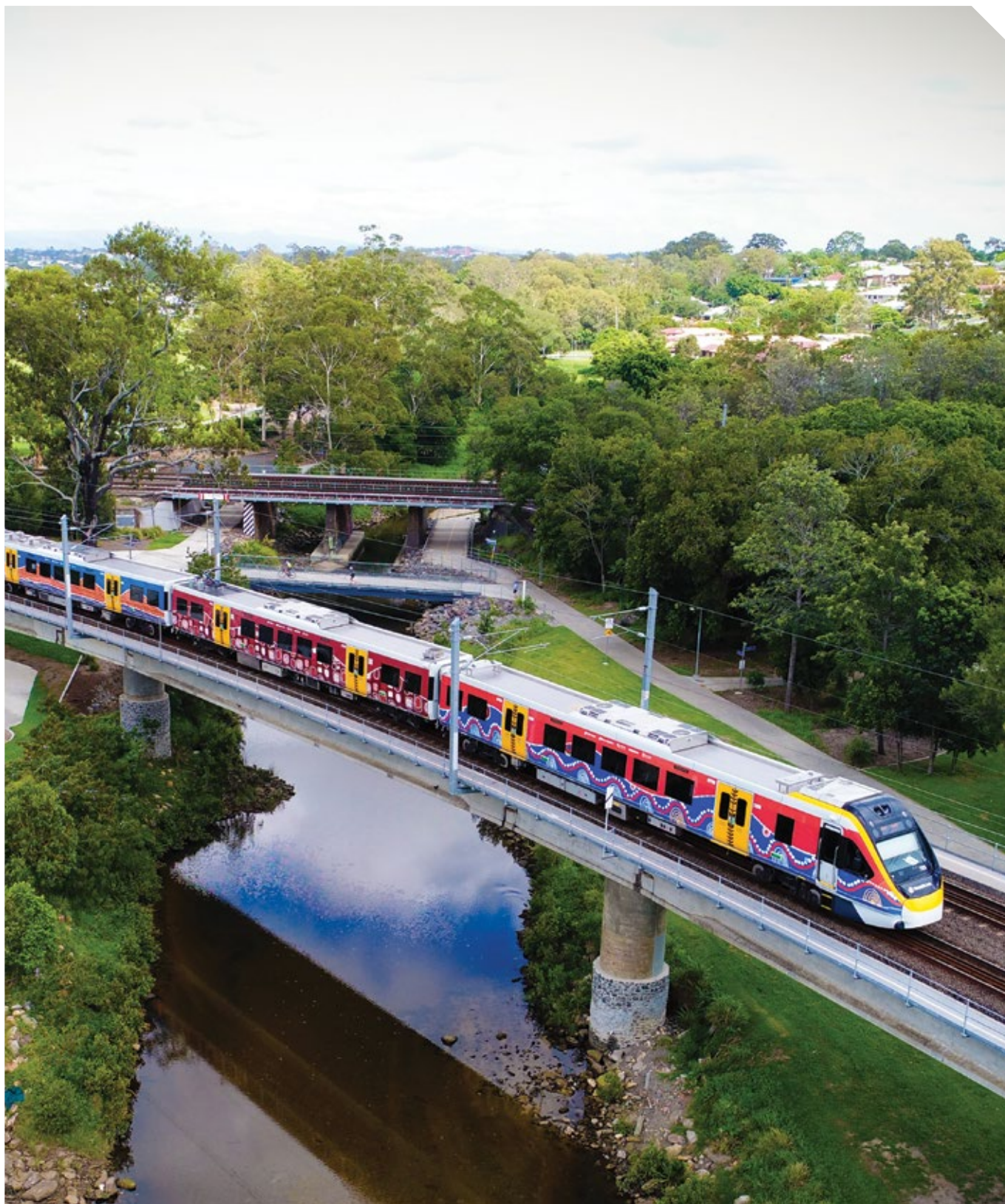
New Generation Rollingstock (Source: Department of Transport and Main Roads)
