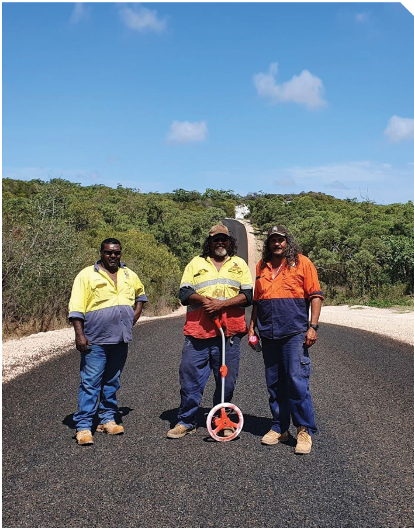
Elim Road, Hopevale (Source: Queensland Reconstruction Authority)
