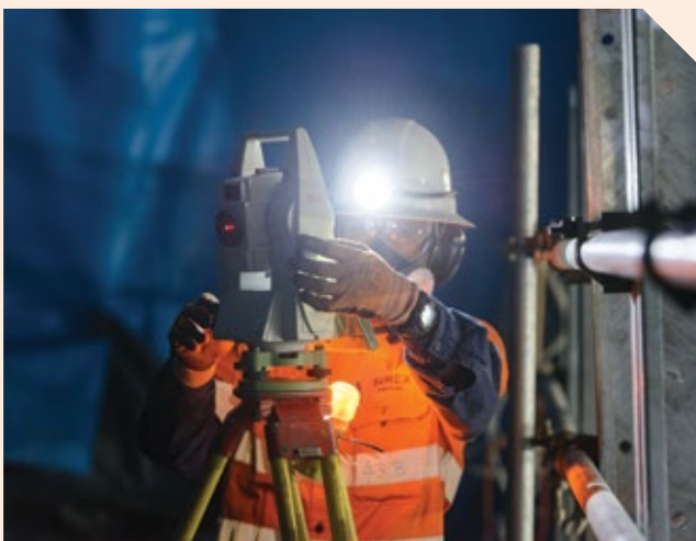
Cross River Rail Construction (Source: Cross River Rail Delivery Authority)
