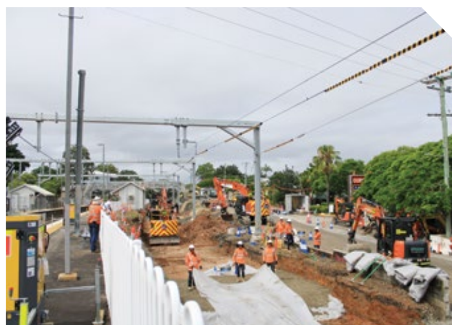
Cross River Rail Construction (Source: Cross River Rail Delivery Authority)
