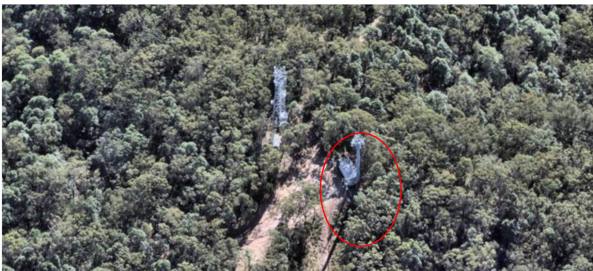
Figure 2: Existing telecommunications facilities within Mooloolah River National Park, Meridian Hill section. The existing monopole upon which Telstra equipment is proposed to be upgraded is shown with red circle. (Source: RFNSA, 2025)
