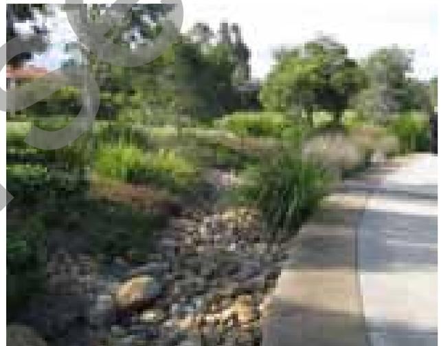
Rock-lined and vegetated bioretention swale
