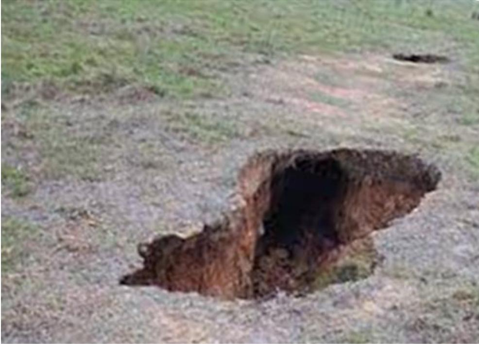
Figure 5 - Example of tunnel erosion or sinkhole over pipeline
