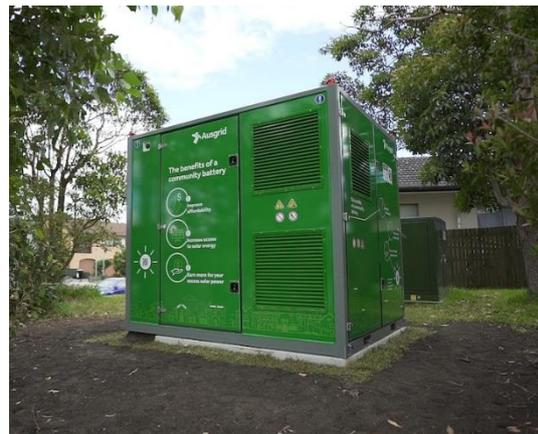
**Figure 2:** A pad mounted battery storage facility,
