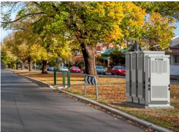
**Figure 1:** A pad mounted battery storage facility,
