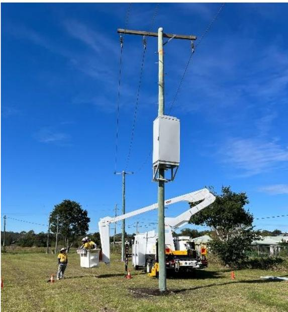
**Figure 4:** A pole mounted battery storage facility,
