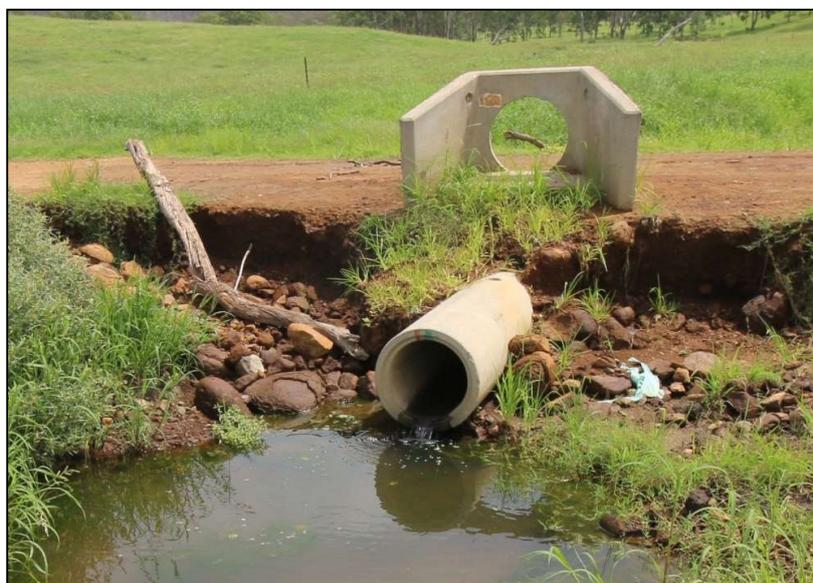
**Figure 5.** The waterway crossing that is acting as a barrier to fish passage.
