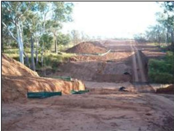
*Figure 8: Erosion controls (berms and sediment fences) at a watercourse crossing. (W. Mathieson)*
