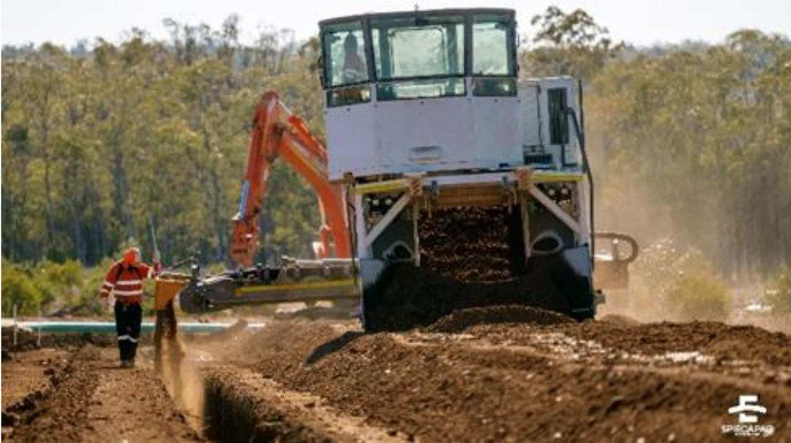
Figure 24: Backfill padding (Spiecapag Australia)
