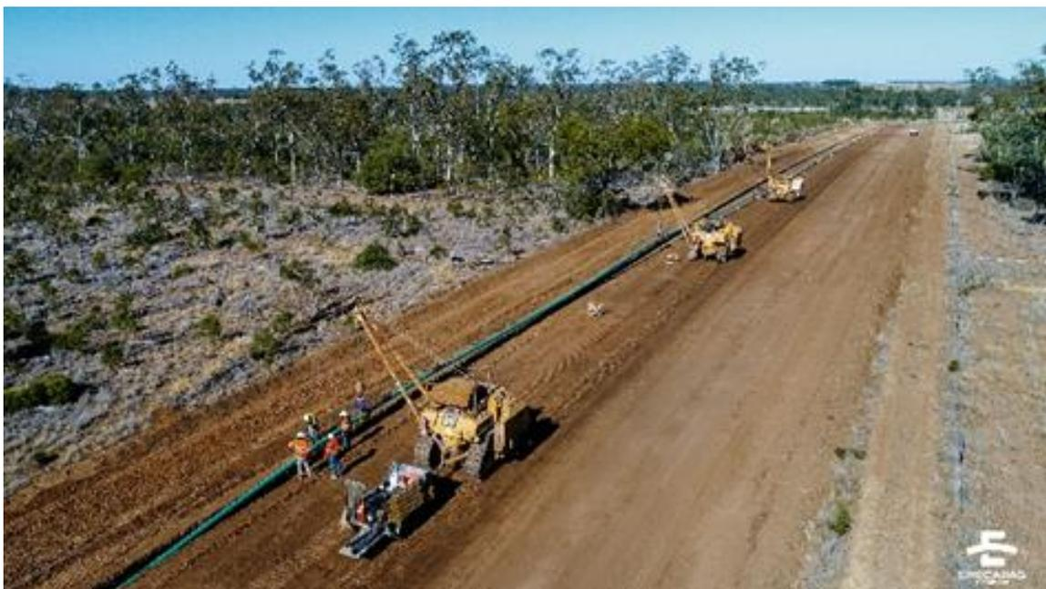
Figure 23: Mainline lower and lay (Spiecapag Australia)
