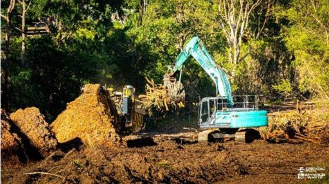
Figure 15: Vegetation clearing and stockpiling (Spiecapag Australia)
