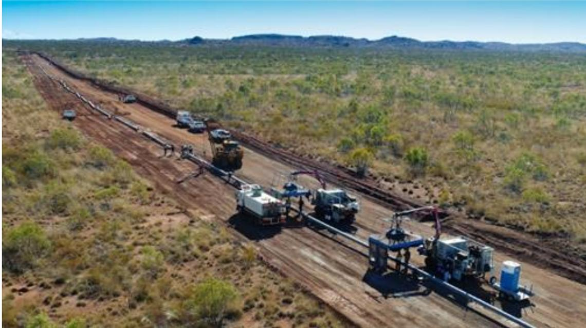
Figure 11: Welding crew operating on the pipeline right of way (Spiecapag Australia)
