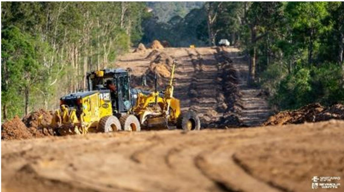
Figure 14: Grader operating during clear and grade (Spiecapag Australia)
