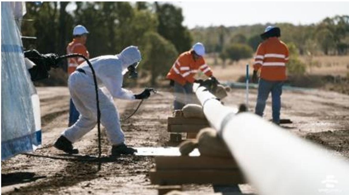
Figure 16: Mainline coating being undertaken (Spiecapag Australia)
