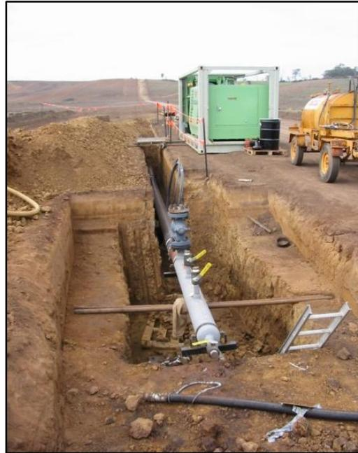
Figure 25: Hydrostatic testing a section of pipeline. (Ecos Consulting)
