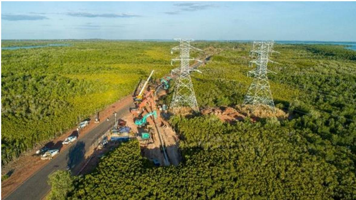
Figure 22: HDD Exit Side Pipe Pull Back operation (Spiecapag Australia)
