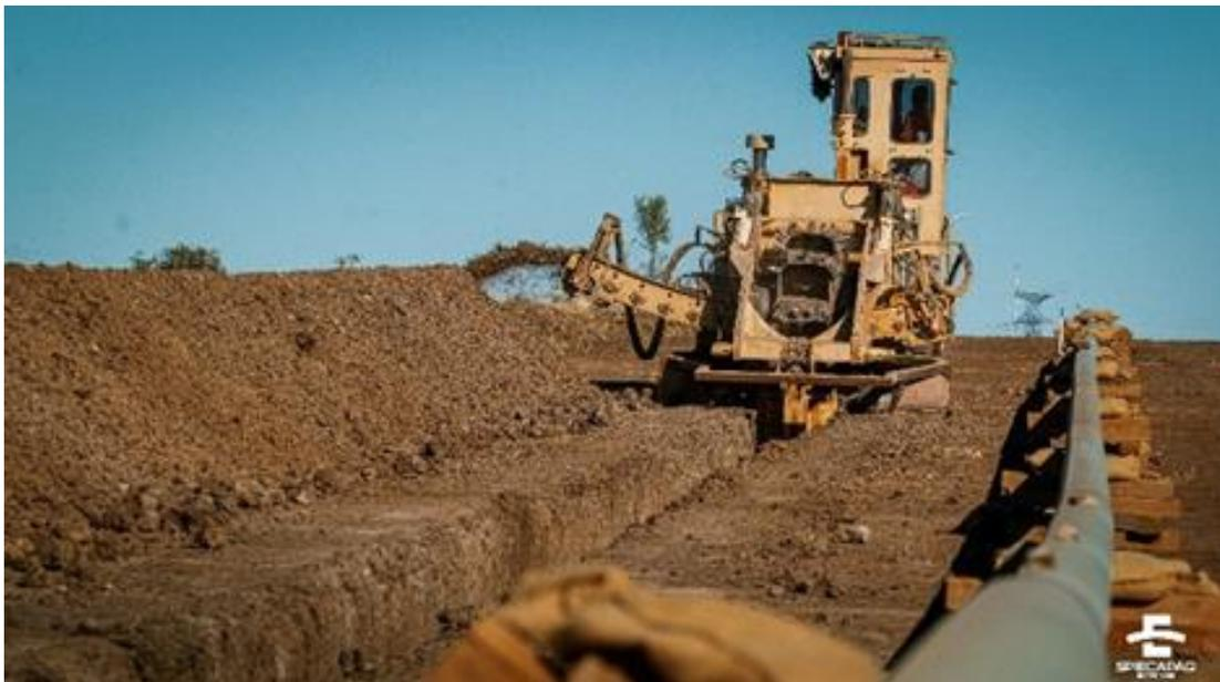
Figure 18: Trenching machine in operation (Spiecapag Australia)
