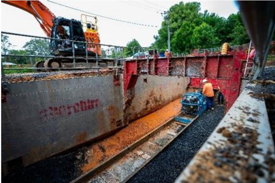
Figure 21: Thrust Boring under highway (Spiecapag Australia)
