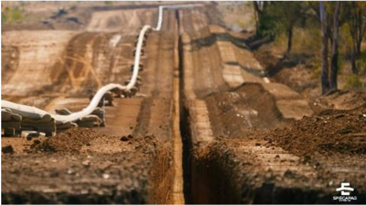
Figure 17: Welded pipeline ready to be lowered into the open trench (Spiecapag Australia)
