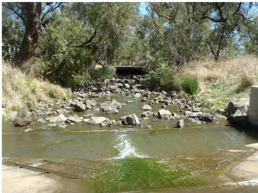
Picture 3-6 Typical rock-ramp fishway structure
