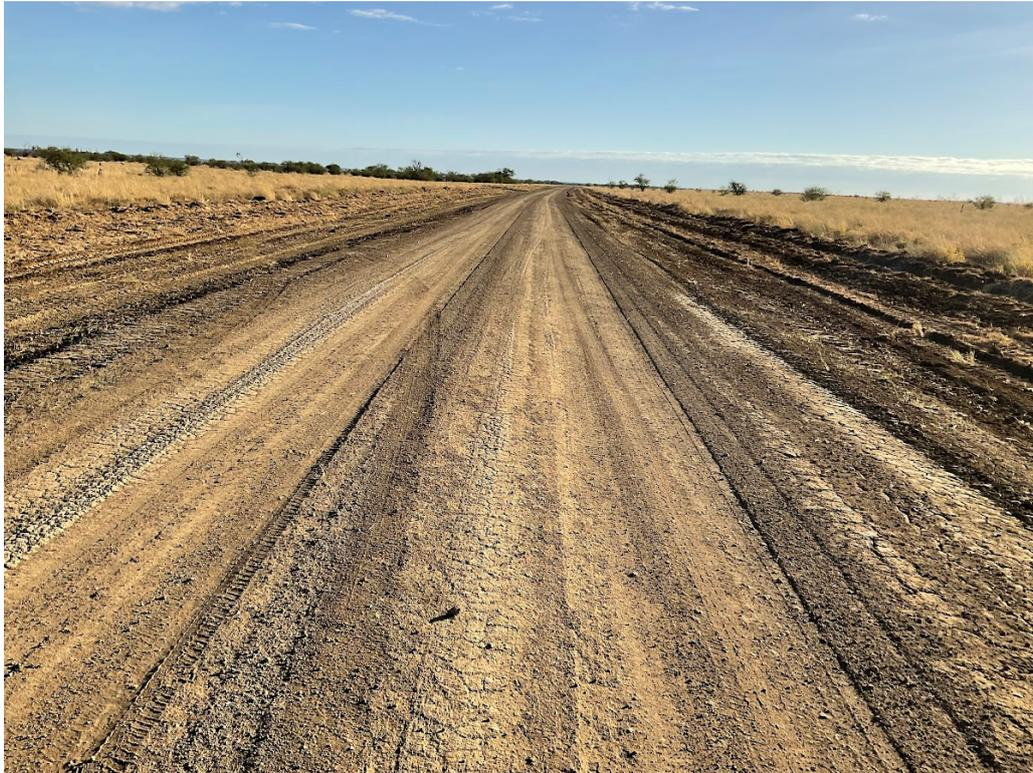
Figure 17: Marathon Stamford Road – Rutting, shoving and cracks
